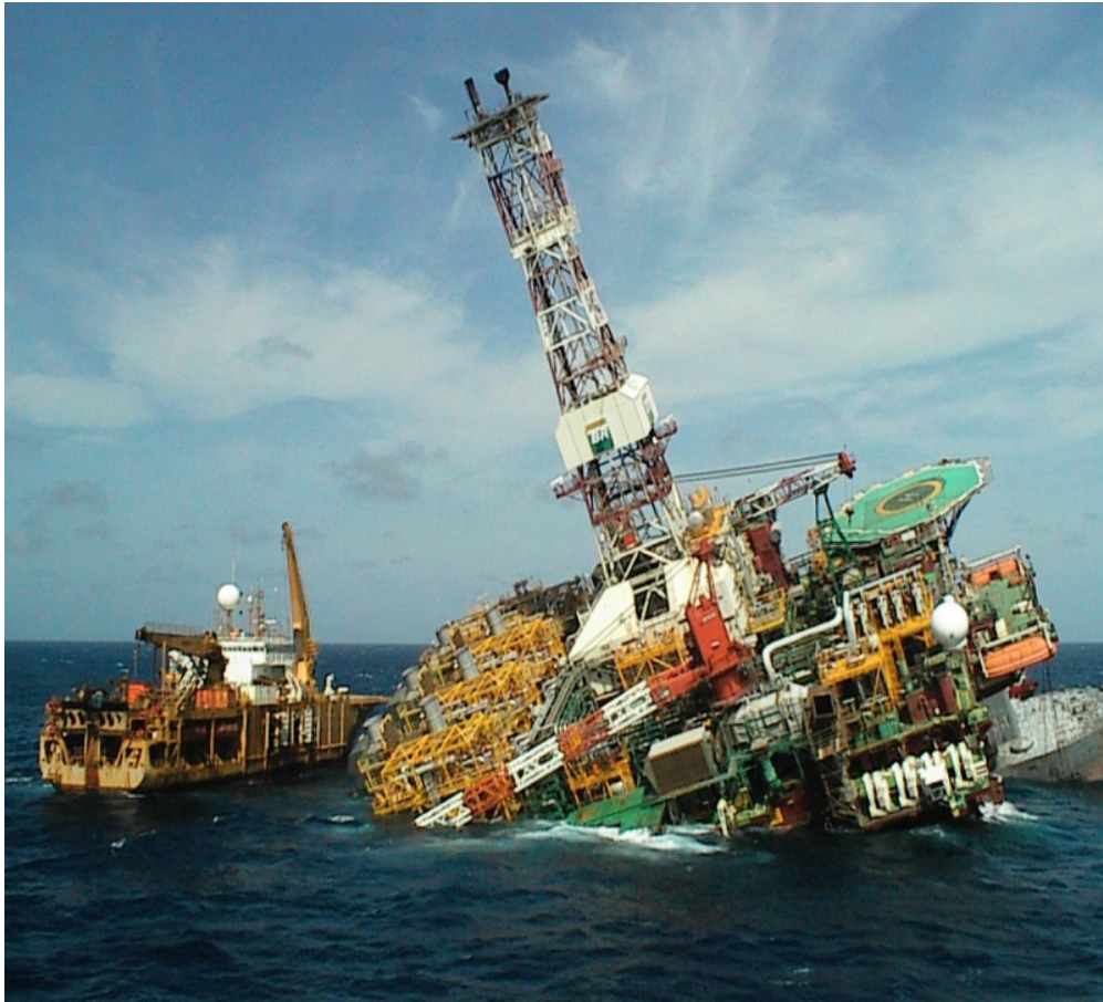
Figure 2.4 The Petrobras P-36 oil platform. P36 No 010 by Richard Collinson
